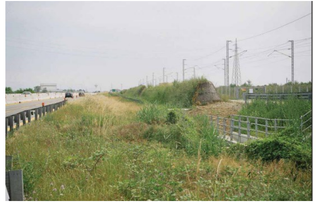
Figure 35. Construction of a noise and anti-glare barrier along the Turin-Milan highway (source: Linee Guida dell'Ambiente e Paesaggio nei settori Infrastrutturali, Ispra 2010)
