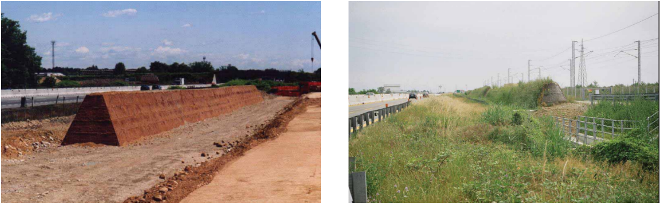
Figure 35. Construction of a noise and anti-glare barrier along the Turin-Milan highway (source: Linee Guida dell'Ambiente e Paesaggio nei settori Infrastrutturali, Ispra 2010)
