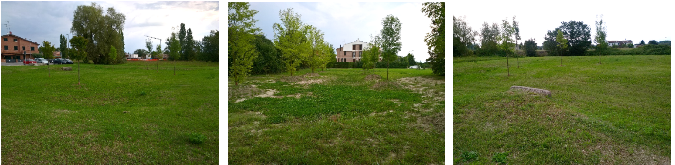
Figure 25. Dry swale with meadows and taller trees as they remain submerged by rains for shorter time, and rear of the emission pipe leading to rainwater discharge pipes. (Photo: Nazaria Marchi, near Ferrara).
